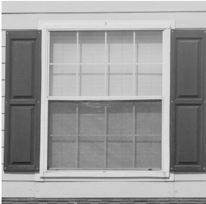
“False” decorative shutters mounted to the wall. Shutters do not match the width of the windows.
