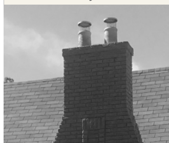
Exposed pre-finished terminations are inappropriate.
