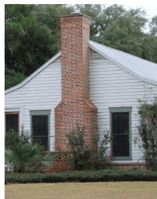
Exposed pre-finished terminations are inappropriate.
