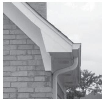
Deep overhangs shall not terminate with an oversized "box" cornice detail or large cornice return.
