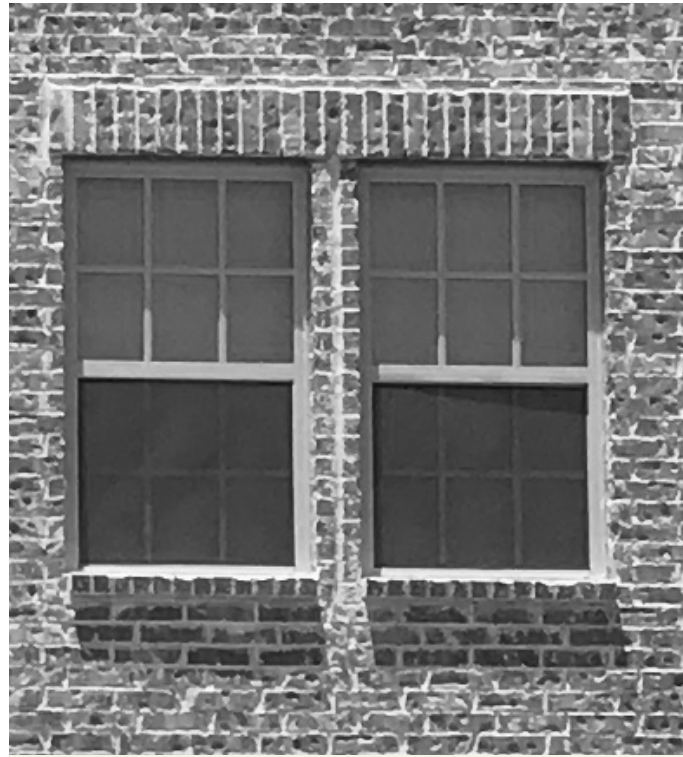
Brick mullion between ganged windows is inappropriate.
