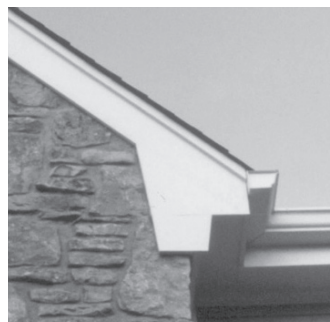
Deep overhangs shall not terminate with an oversized "box" cornice detail or large cornice return.
