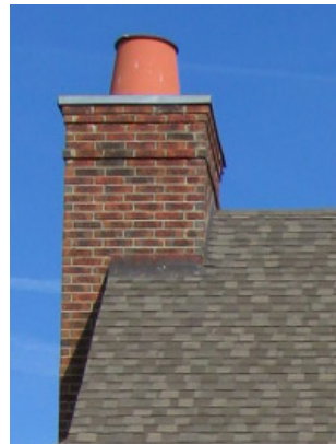
Lap siding shall not be used as a finish material for a chimney.
