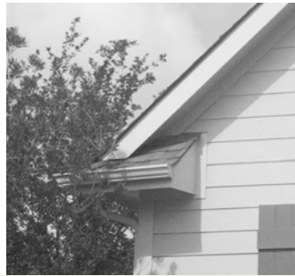
Roof pitch of cornice returns is too steep.
