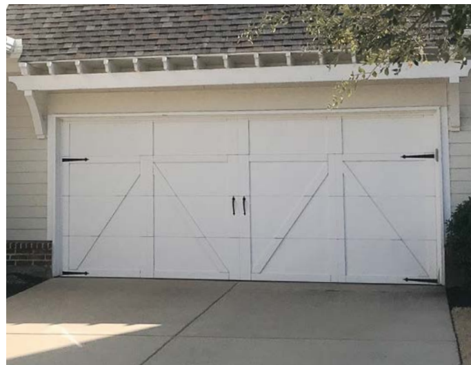
Stamped "false panel" steel doors are not appropriate.
