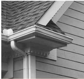
Roof pitch of cornice returns is too steep.
