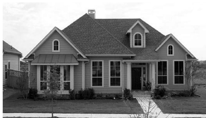
The complex roof elements, the steep pitched roof at cornice returns, the over scaled bay roof, the ill-proportioned dormer and the front entry details are all inappropriate both individually and collectively.
