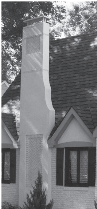
Chimney depth does not reflect traditional masonry construction.
