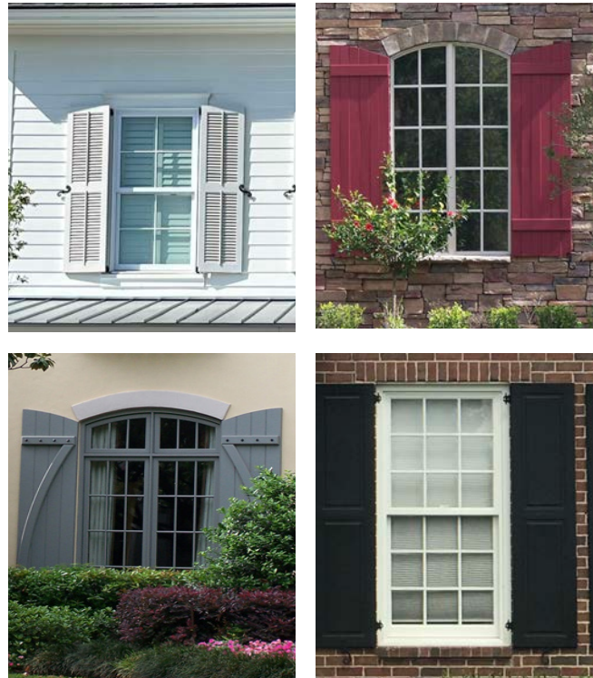
“False” decorative shutters mounted to the wall. Shutters do not match the width of the windows.
