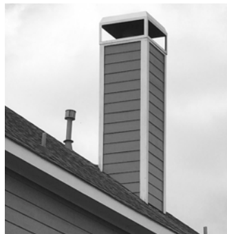
Lap siding shall not be used as a finish material for a chimney.
